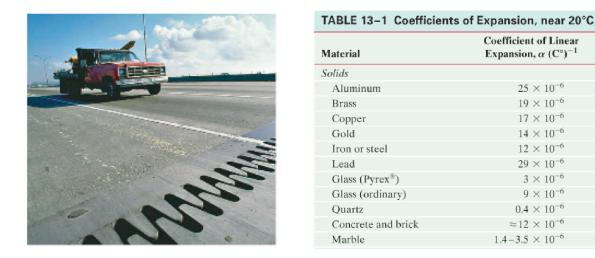
Example: a bridge deck is made of concrete slabs that are 10.0 meters long at 20°C. How wide should the expansion cracks between the slabs be (at 20°C) to prevent buckling if the range of temperatures is  $-20^{\circ}$ C to  $+40^{\circ}$ C? Use  $\alpha = 12 \times 10^{-6}/^{\circ}$ C for the coefficient of linear expansion of concrete. Answer: 2.4 mm.
